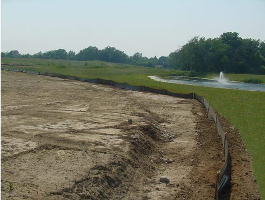
Silt fence installed correctly
