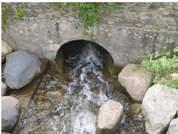
Inlet pipe under private drive crossing (On South side, looking north)
