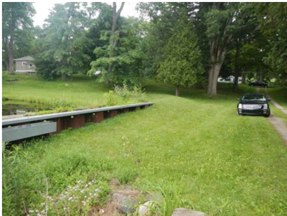
East embankment (Looking east)
