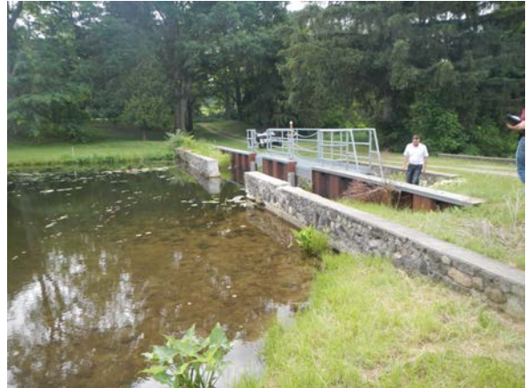
Upstream side of structure (Looking east)
