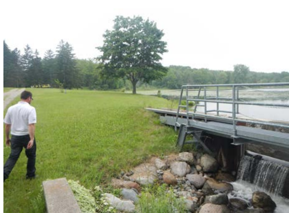
West embankment (Looking west)
