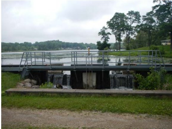
Downstream side of structure (Looking north)
