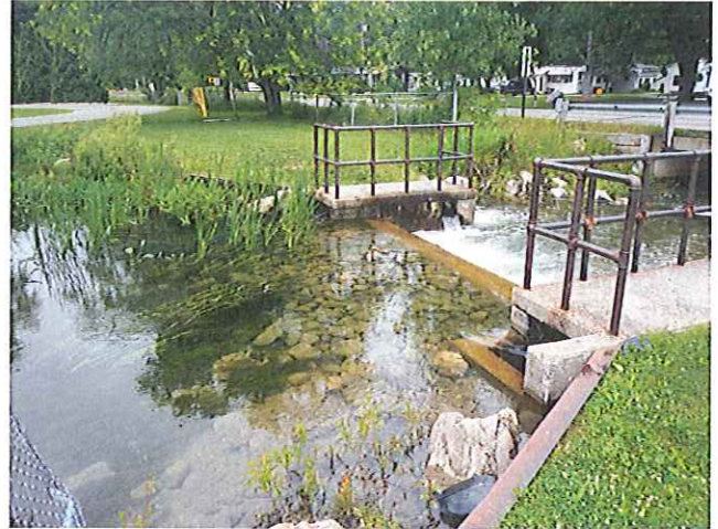
South Side of Dam
