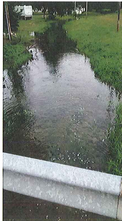
Looking downstream at outlet channel
