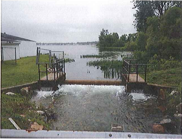
North Side of Dam
