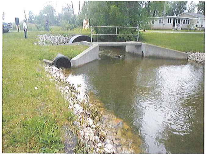
East Side of Posey Lake Dam
