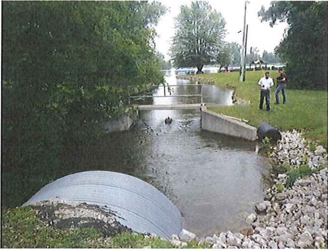
West Side of Posey Lake Dam
