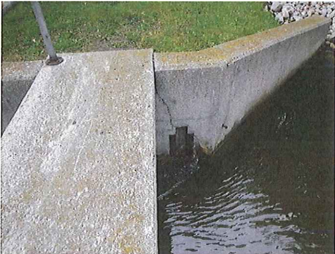
Crack-Northeast Side
