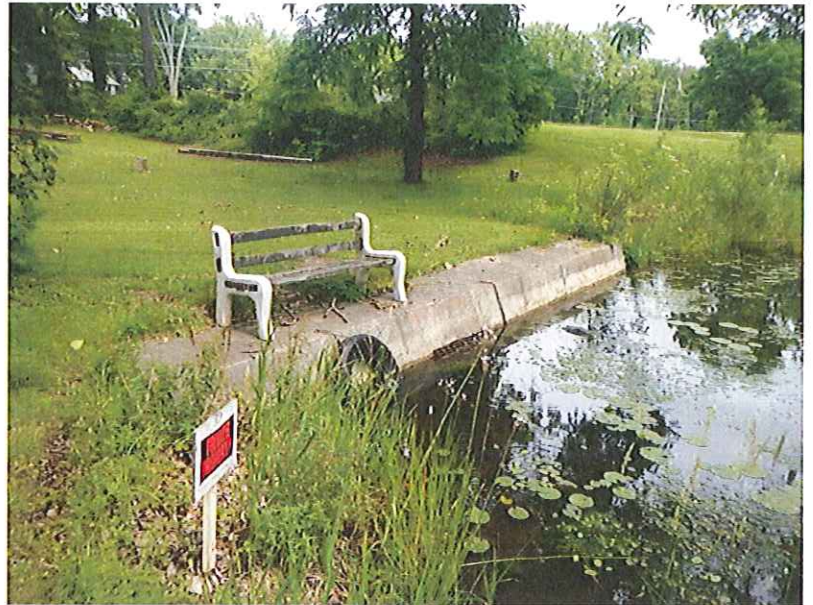
South Side of US-12 Structure
