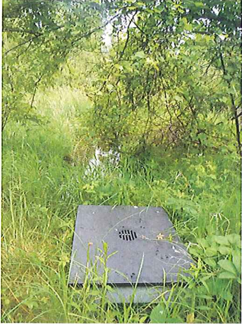
North Side US-12 Control Structure
